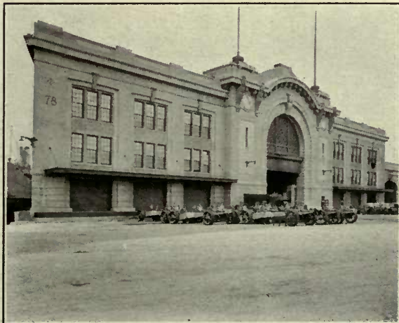
Municipal Pier No. 78, Philadelphia, Pa. Snare & Triest Co., General Contractors
